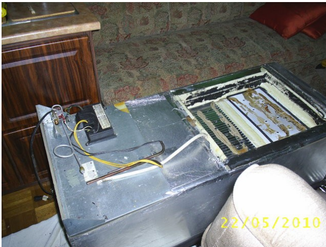
Ready for the new unit
